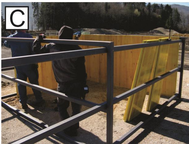
Figure S2 Different stages of a field construction of lysimeters: Metal rod support structure (A) and the same structure placed at the final location of lysimeters (B), installation of an internal box structure, made from water resistant formwork plates (C), and the bottom-up view on the finalized structure of the box lysimeters, with a lysimeter percolate collection tank placed in front (D).
